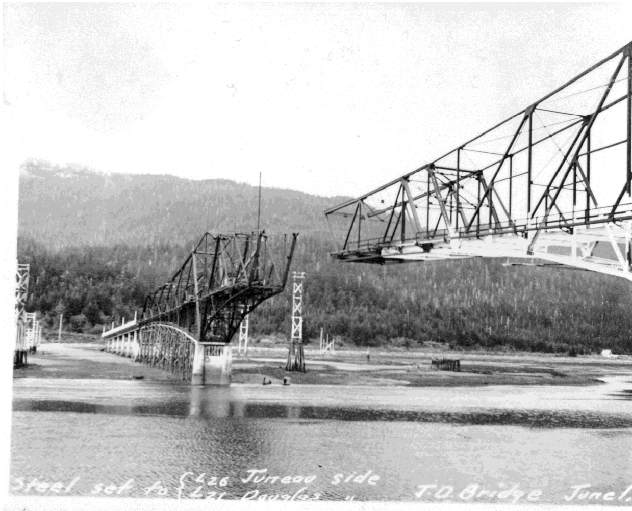
Juneau-Douglas Bridge Construction, circa 1935
