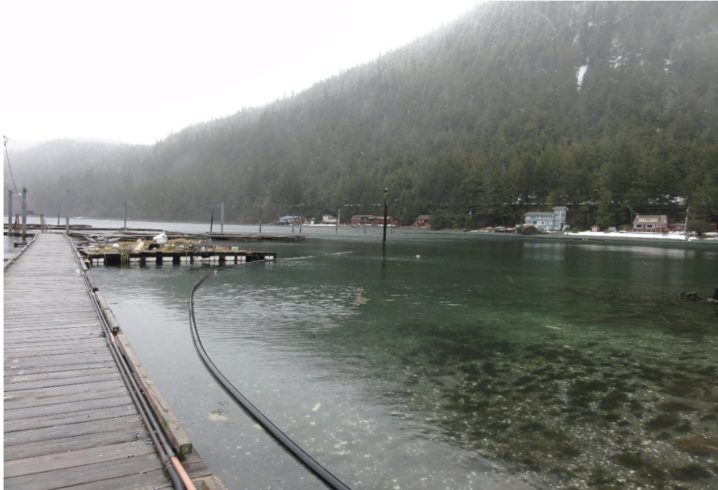
PHOTO 3– Looking in a Northeast direction from a permanent fixed float toward subject detached tidelands. (041221(100))
