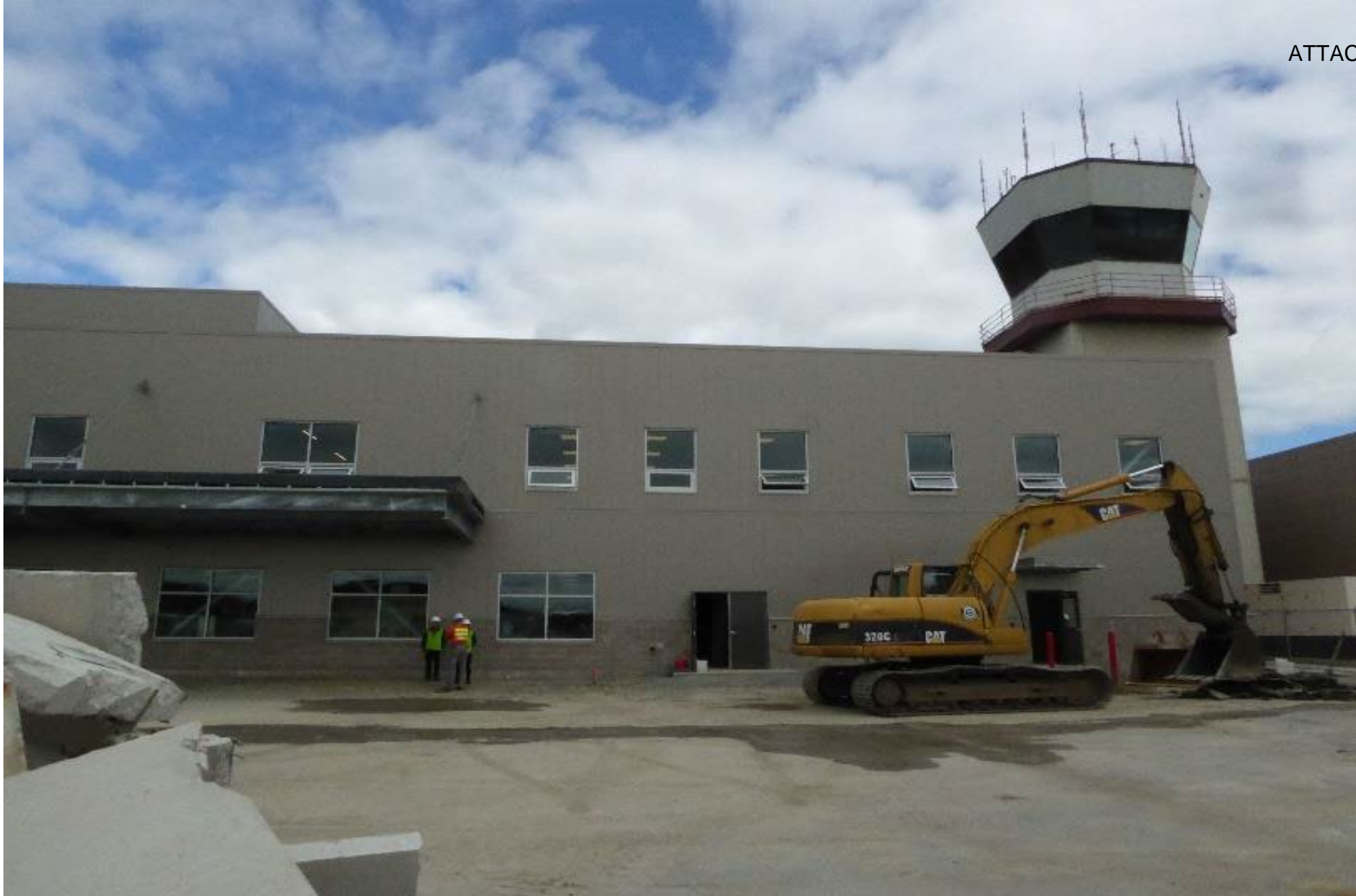
Excavation for ramp paving along west (airfield/ramp) side of building.
