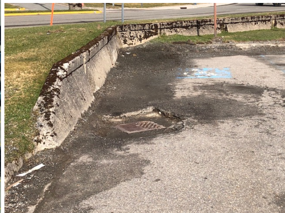
Long term parking lot failing vault
