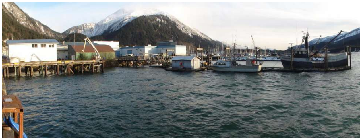
Photo showing White Crain Dock photo left with main float and pier photo center. Note ramp and float photo right.
