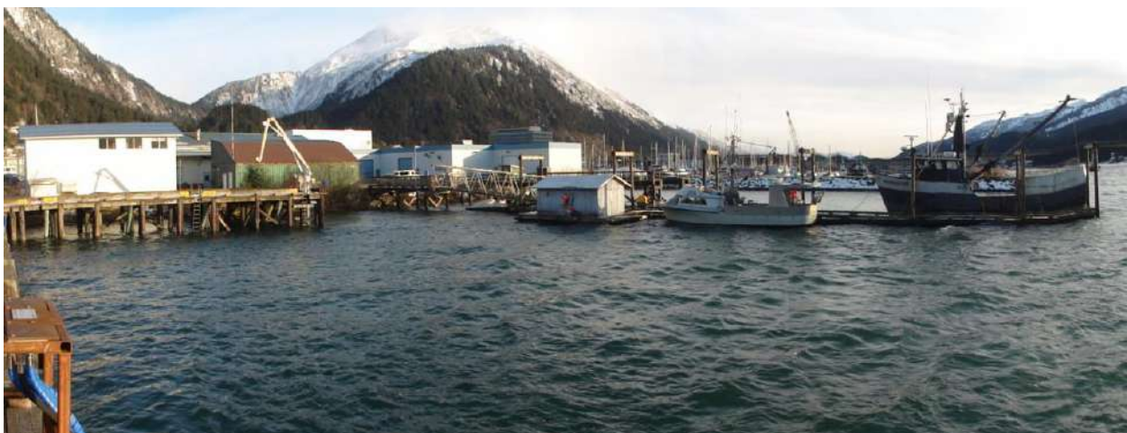
Photo showing White Crane Dock photo left with main float and pier photo center. Note ramp and float photo right.
