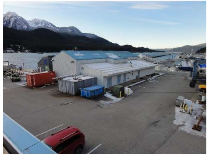
Figure 3.8 – Welding lab as viewed from the roof of the TEC Building.
