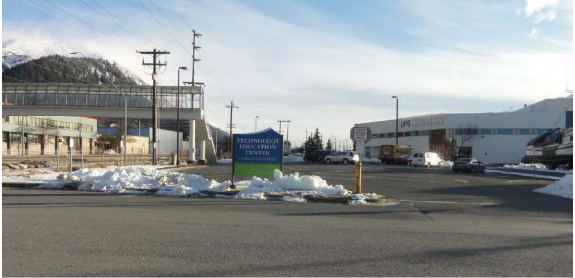
View of subject as it fronts Egan Drive looking in a southerly direction.
