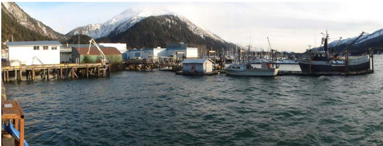
Photo showing White Crane Dock photo left with main float and pier photo center. Note ramp and float photo right.
