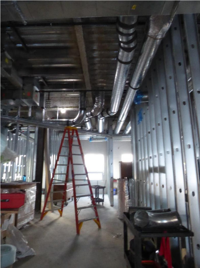
View into airport admin reception office from balcony.
