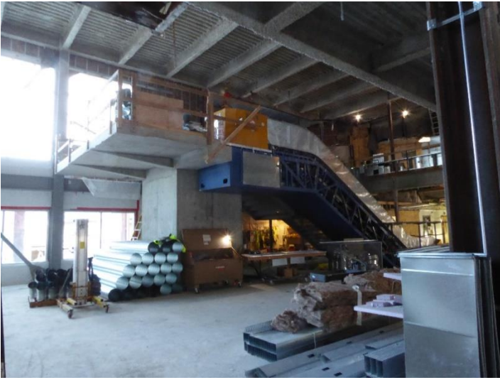
Stair tower with escalator installed.
