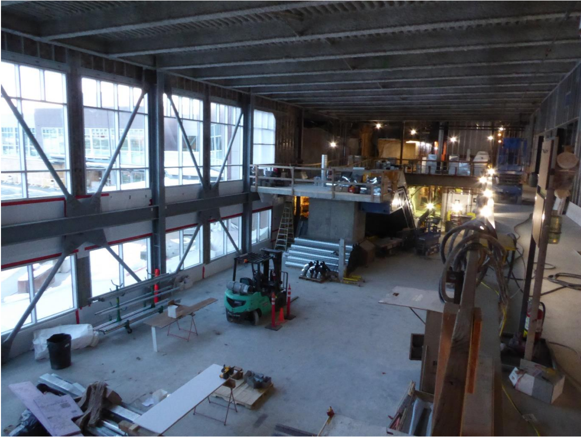
Regional air carrier seating area viewed from 2 nd floor balcony.
