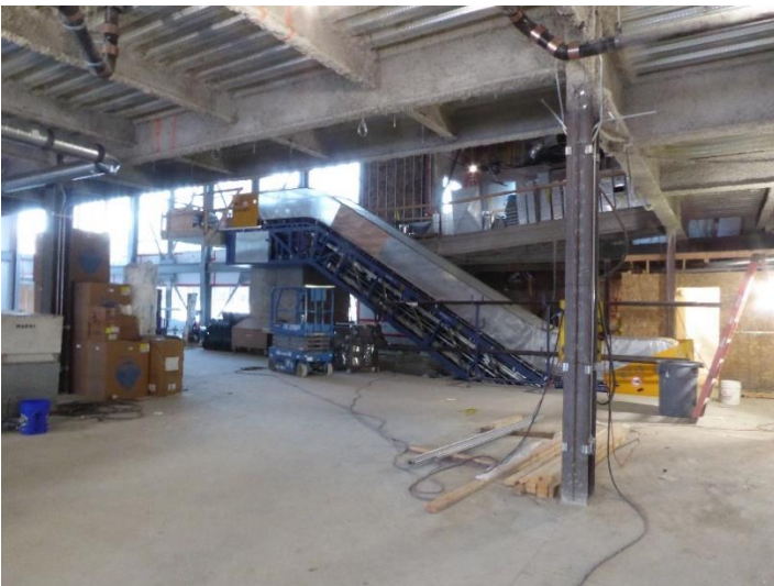
Escalator & ramp viewed from west seating area.
