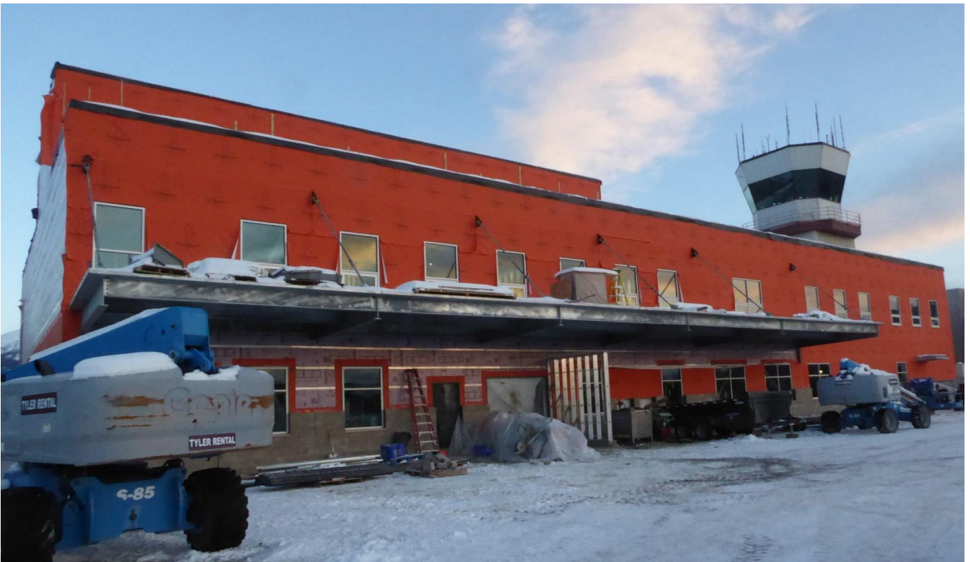
West elevation with Gate 1 located adjacent metal framed wing wall.
