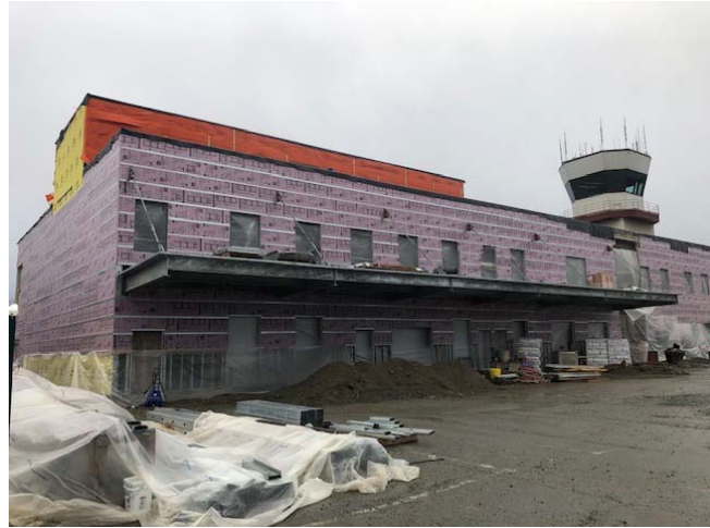
Photo 02: Airside of the terminal.
