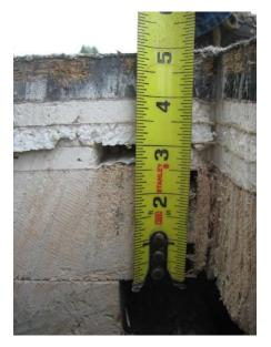
8. The original roof assembly was no better than that addition with the following composition: 3x wood deck, ½ " polystyrene insulation, 1" fiberboard, ½ " built-up roof, ½" OSB, and then new roof membrane. Unfortunately, the roof appears to be in decent shape despite debris and ponding noted in earlier report and probably has 5-10 years of useful life before replacement should be contemplated. However, this time frame may be shortened if energy prices continue to climb.
