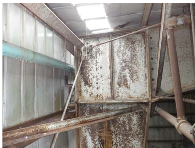
TYPICAL BRACE TO COLUMN CONNECTION
