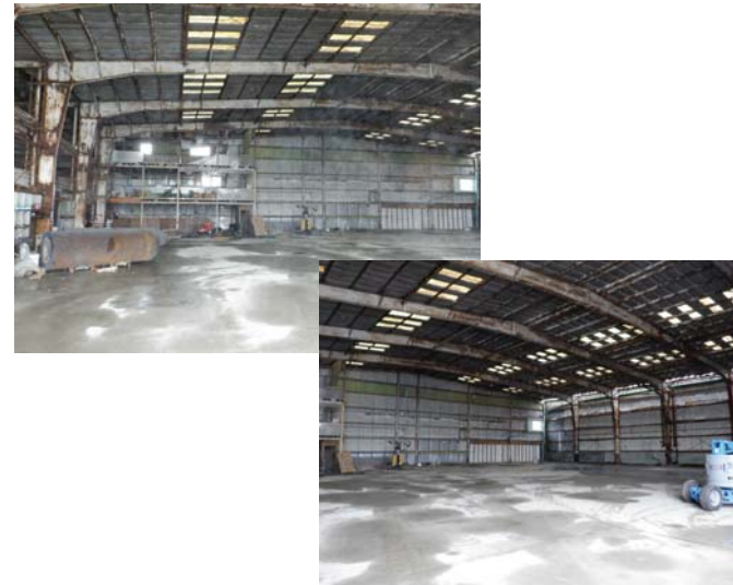
OVERALL BUILDING - INTERIOR
