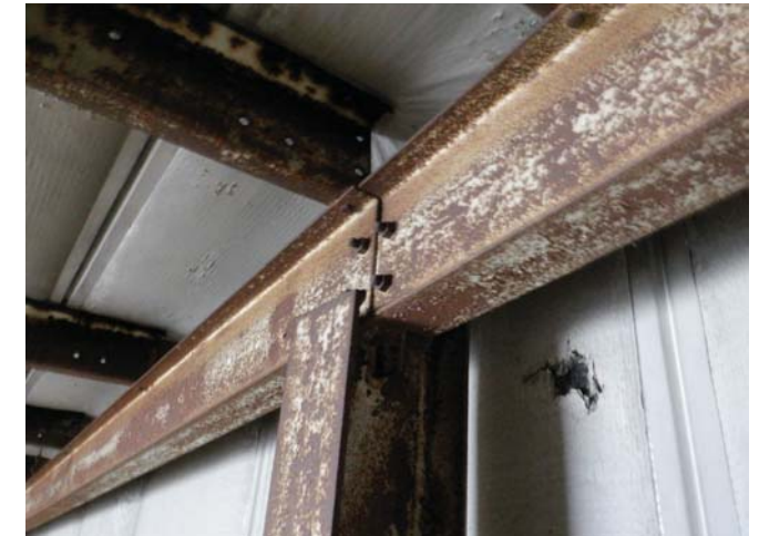
TYPICAL ENDWALL BEAM SUPPORT
