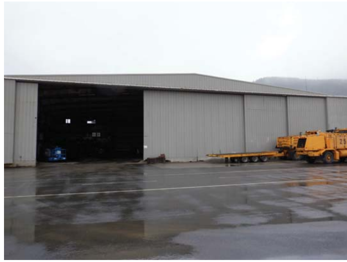
OVERALL BUILDING - SECURED SIDE
