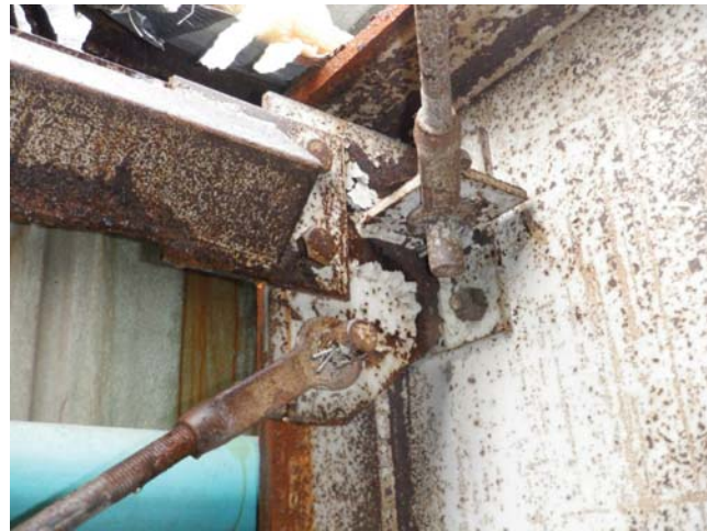
TYPICAL BRACE TO COLUMN CONNECTION
