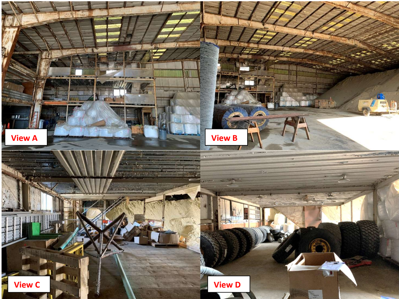
FIGURE 2. Sand Storage Building, Views A-D
