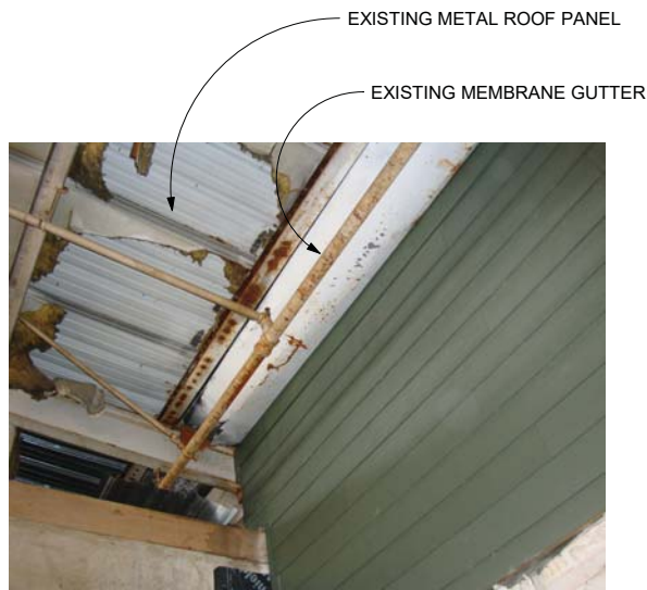
5 PHOTO OF BOTTOM OF EXISTING ROOF TO REMAIN NTS
