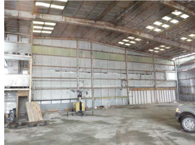
TYPICAL END WALL FRAMING
