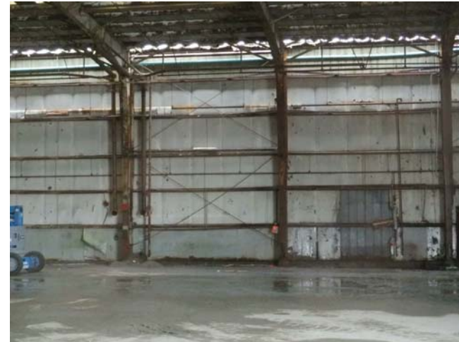
TYPICAL BRACED FRAME BAY ALONG SHARED WALL
