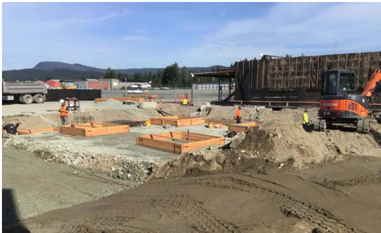
From airside, looking northeasterly into work area.
