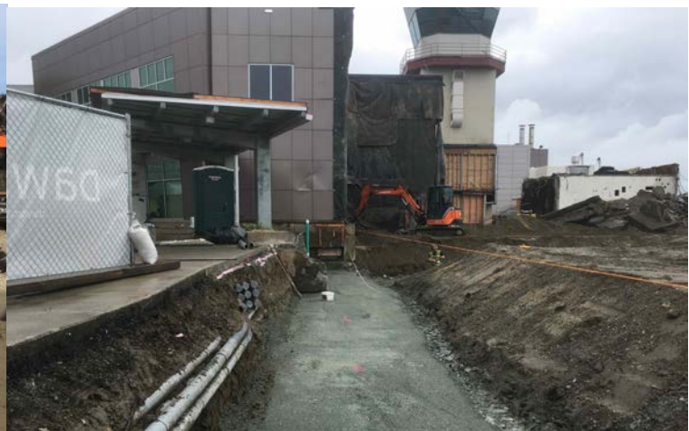
Along Shell Simmons Drive, looking westerly toward terminal.
