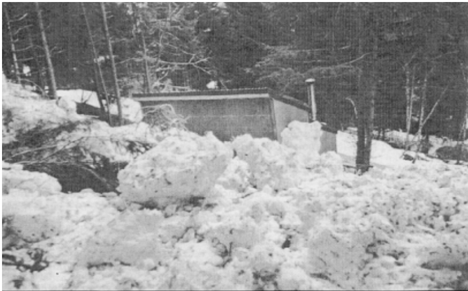
White Subdivision residence after avalanche of February 20, 1985. Only the second story is visible above the avalanche debris. Photo by Doug Fesler.
