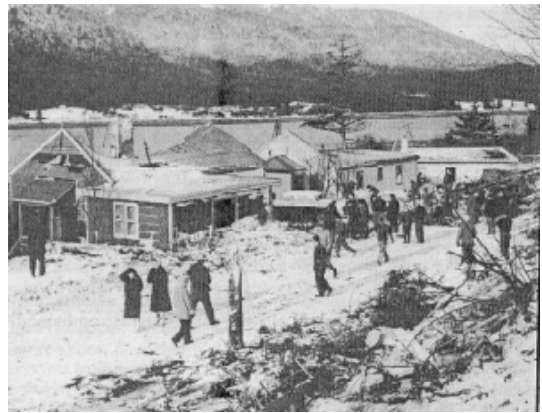
Residents examine debris and powderblast damage from March 22, 1962 Behrends Avenue avalanche.
