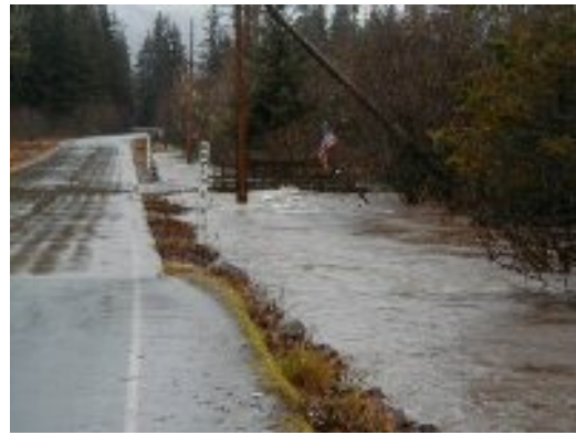
Montana Creek flooding.
