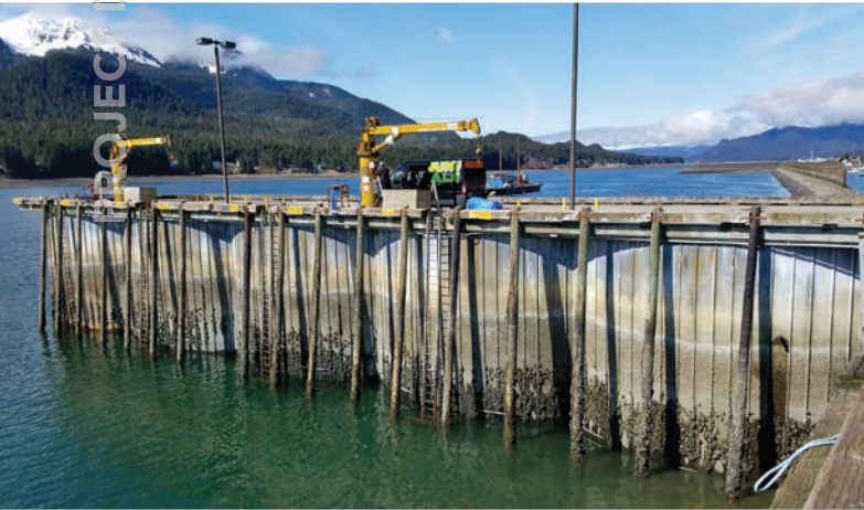
Figure 5 – (above) Fender pile and bull rail construction on south side of existing crane dock; (right) Existing Crane; (below) North side of the rubble mound breakwater where the new dock face will be constructed.
