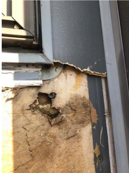
Figure 4: Saturated Gypsum
