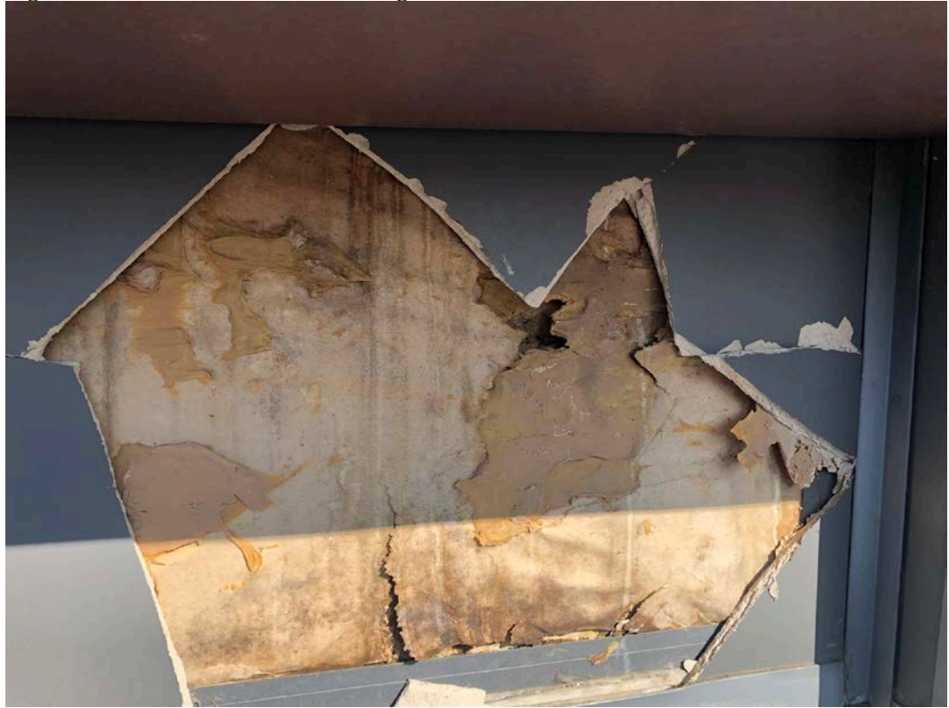
Figure 7: Sealant failure at window
