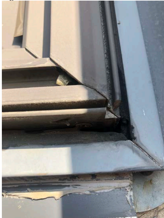
Figure 7: Sealant failure at window
