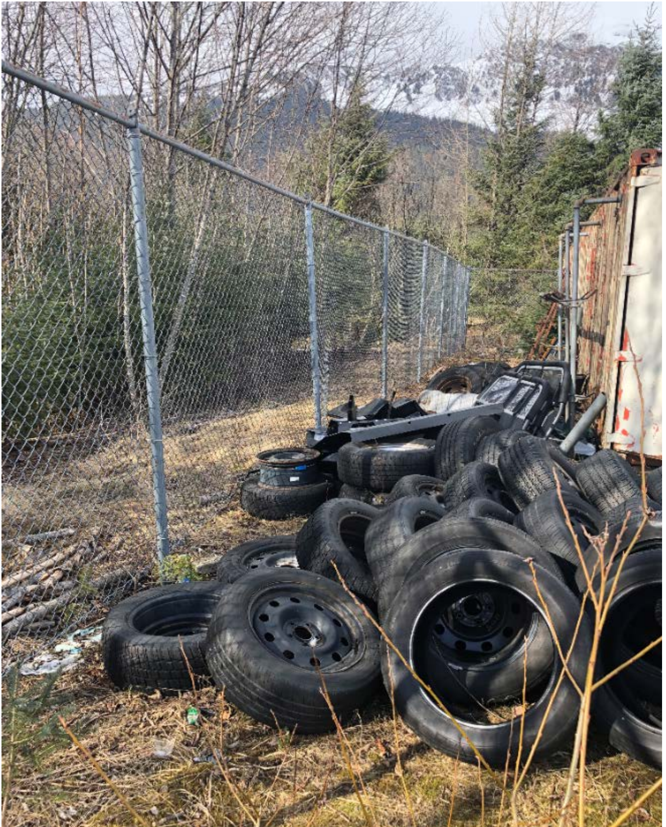
JPD will remove the Tires and Misc. Equipment pictured prior to fence reinforcement installation.
