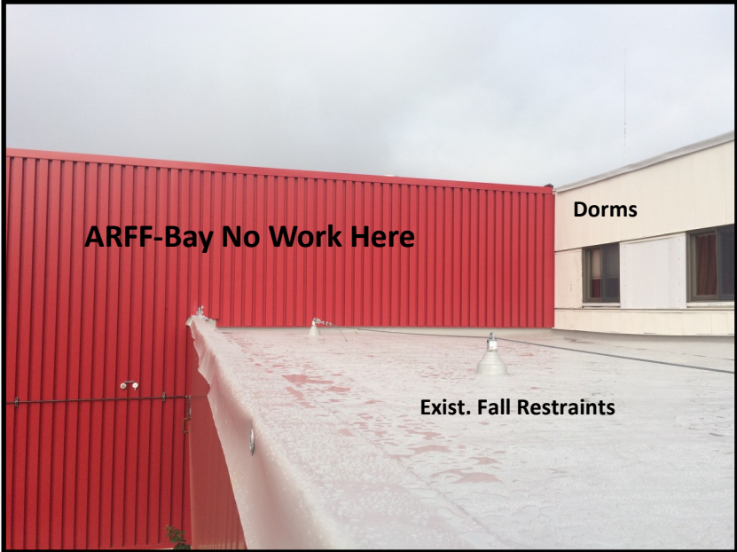
2017- Roof Replacement project. PVC roofing at parapet, typ. Detail before flashing.
