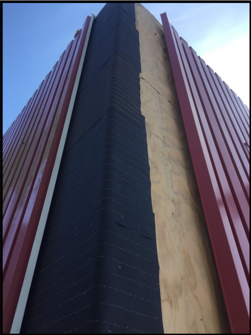
Exist. Wall Assb'y—NE Corner of 2018 rot repair.
