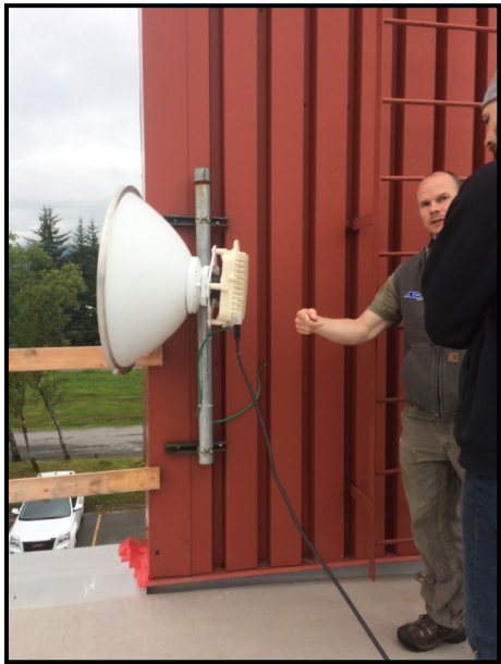
Microwave dish on Hose Tower—Remove & Reinstall. Coord. W/Proj. Mgr.
