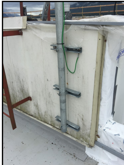
Uni-Strut mounting detail (Same dish)
