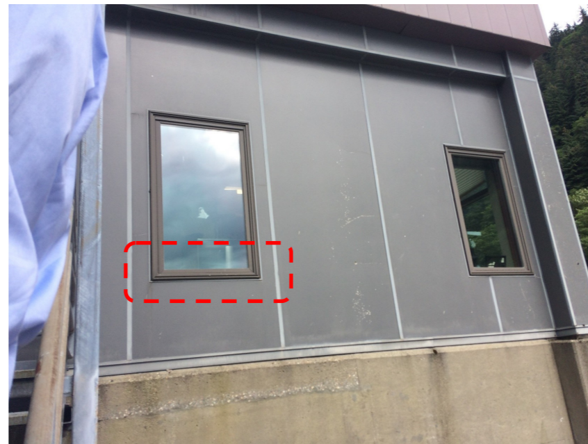
SOUTH FAÇADE (FACING DOWN CHANNEL)
