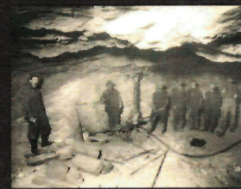
Underground lode mining in a "breadth mine" 1908. The process was called drift, blast and block. Miners first drilled holes in the rock with a large jack-leg rotary drill, and then packed it with explosives. After the blast, they trucked out the ore and sent it to the mill.
