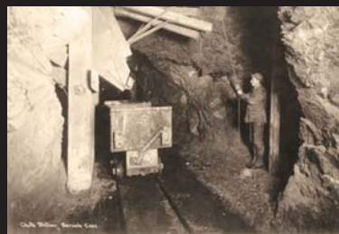
Perseverance Mine underground chute station ALASKA STATE LIBRARY, HISTORICAL COLLECTIONS, WINTER AND POND, ASLP87-1422
