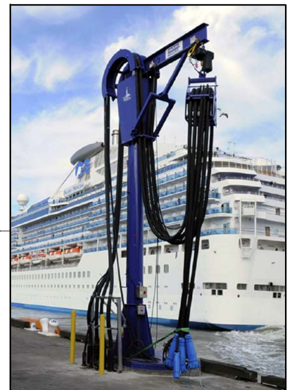
CABLE POSITIONING DEVICE w/ 15' EXTENDABLE BOOM (PHOTO USED WITH PERMISSION FROM COCHRAN MARINE.)
