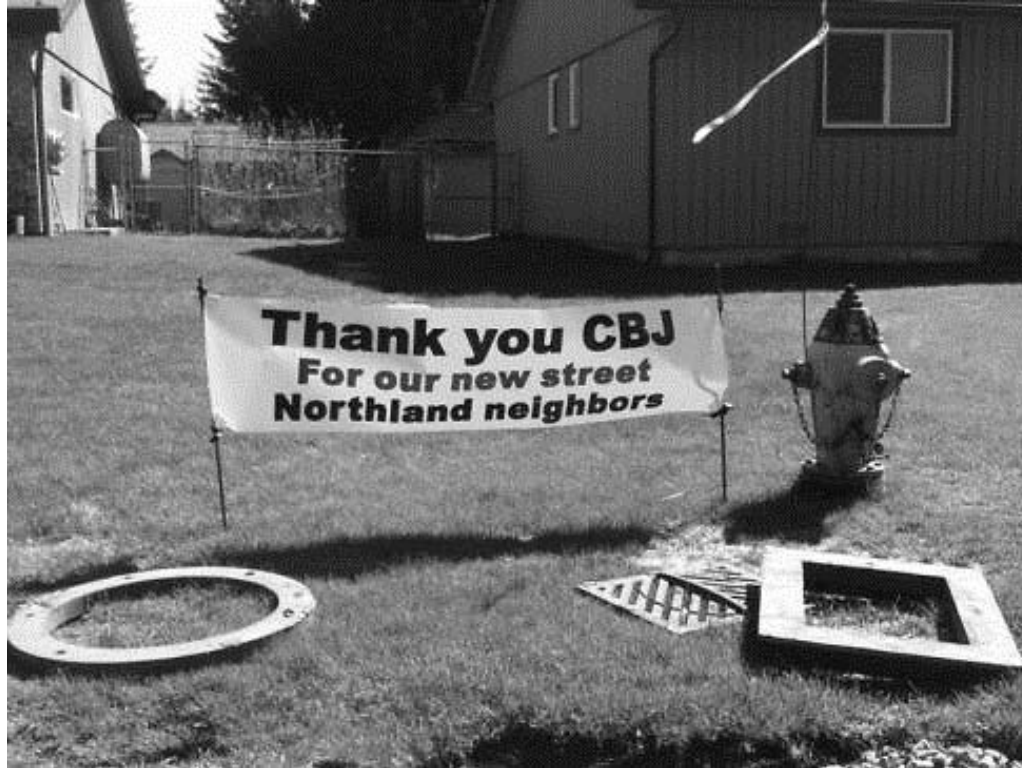
Northland Street Reconstruction
