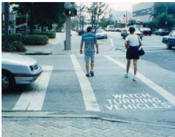
Figure 22 Warning Striping for Turning Vehicles
