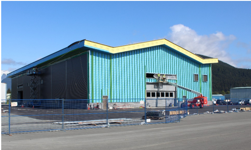
Sand/Chemical Building from SW corner.
