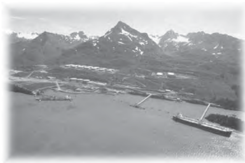
Valdez oil terminal
