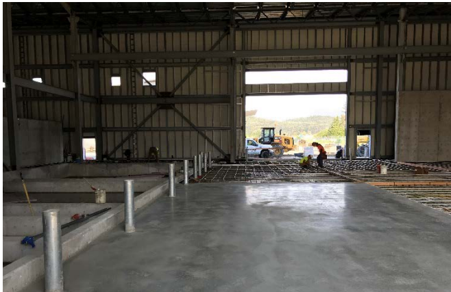
Sand/Chemical Building interior concrete slabs
