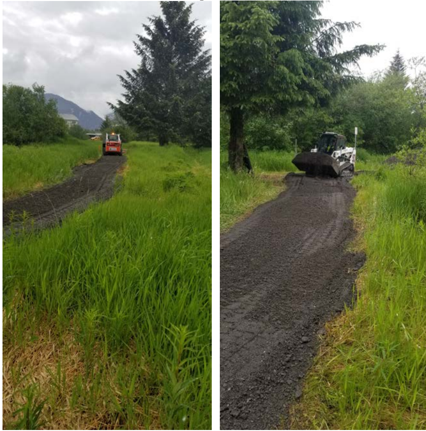
Jordan Creek trail widened/improved
