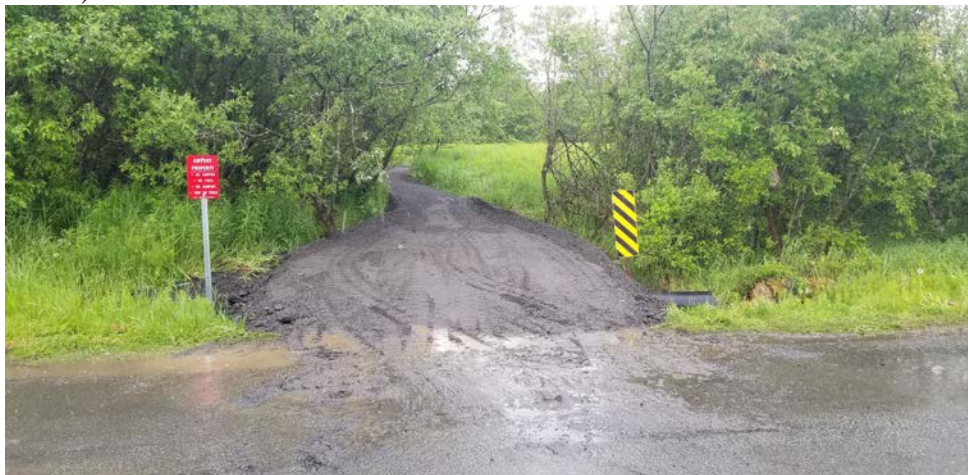
Jordan Creek trail widened/improved off Alpine (note: removed temporary ROW access)
