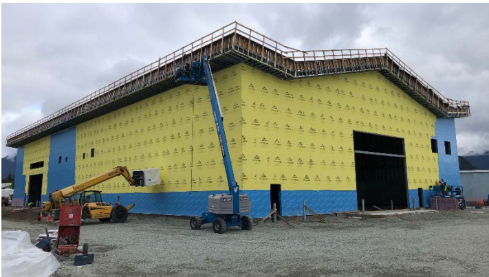
Sand/Chemical Building from SW Corner
