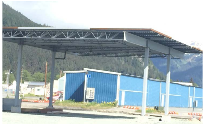
Fueling Station Canopy
