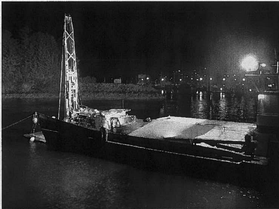
Photo 1. Drilling operation at night in the harbor.
