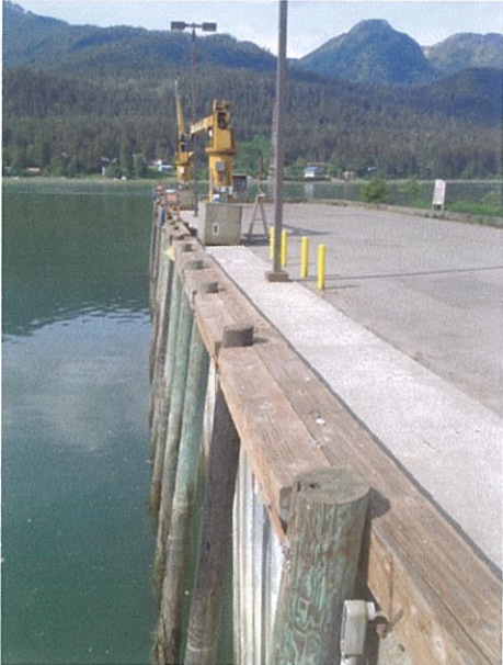
Detail of Fender Piles & Bull Rail
