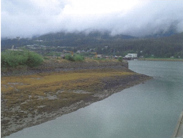
North Side Of Rubble Mound Breakwater – New Dock Face Will Be Built Here
