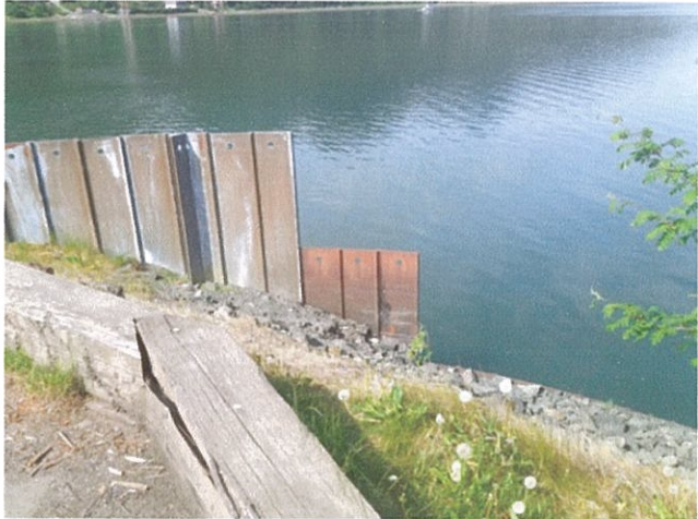
End of Sheet Pile Cell – New Construction Will Connect To This
