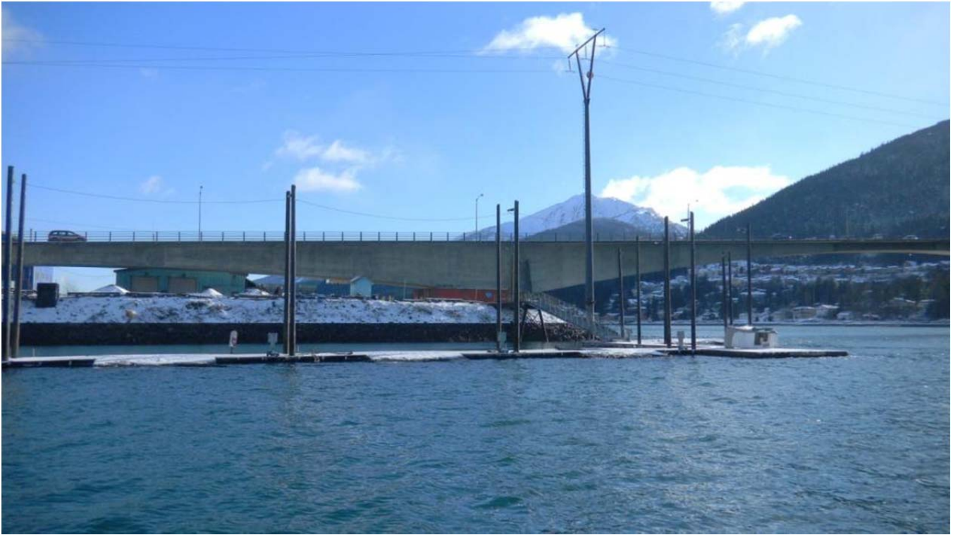
View of existing float plane dock at the Douglas Bridge.
