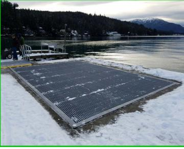
Coverings: Docks & Harbors is committed to providing safe and secure facilities with a high level of customer satisfaction. We recently completed a pilot project to validate "decking over" the openings on the Statter Breakwater. We will evaluate the success of the fiber grates over the next months to determine future construction plans.
