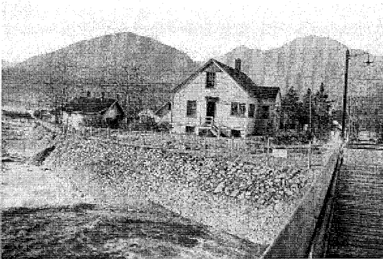
Gold Creek after log and rock cribbing placed to control flooding, 1943 Courtesy of the Green Family
