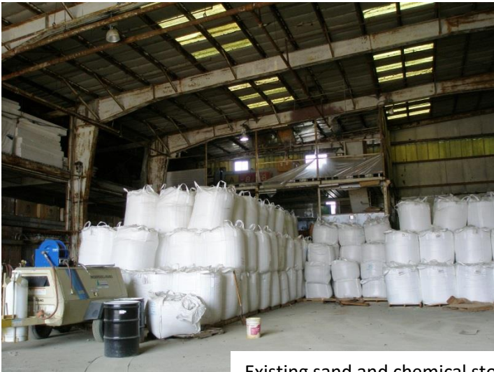
Existing sand and chemical storage building.
