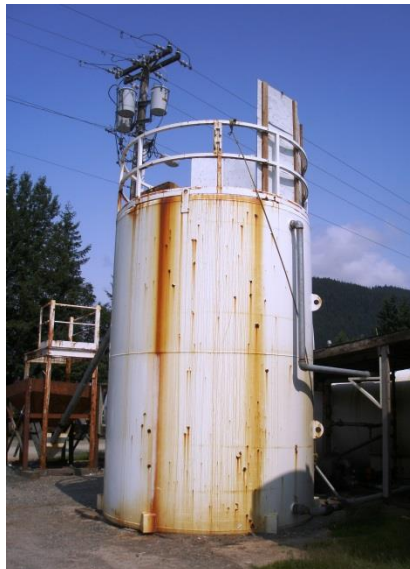
Existing chemical mixing tank & mixing platform.
