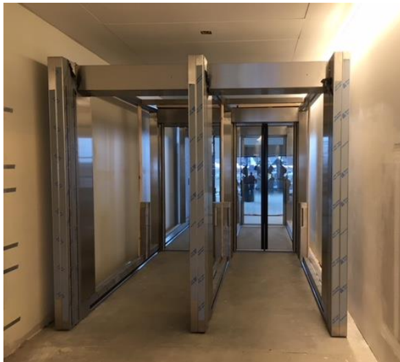
Automated exit lane under construction at Paine Field Terminal.
