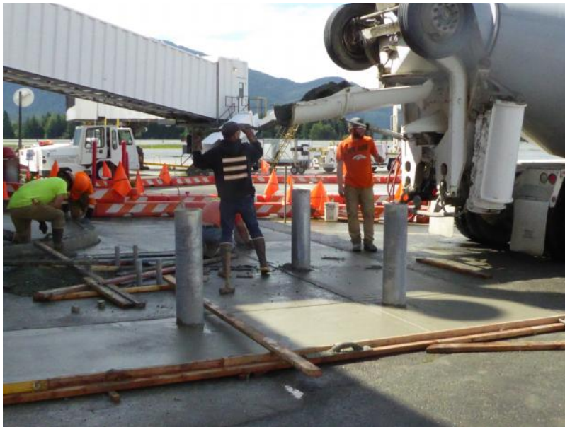
Concrete Placement at Gate 2 Passenger Boarding Bridge.
