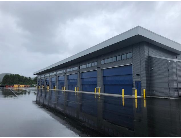
SREB exterior doors painted, and east wall of maintenance bay receives siding (wash bay reclamation pit formwork at right).
