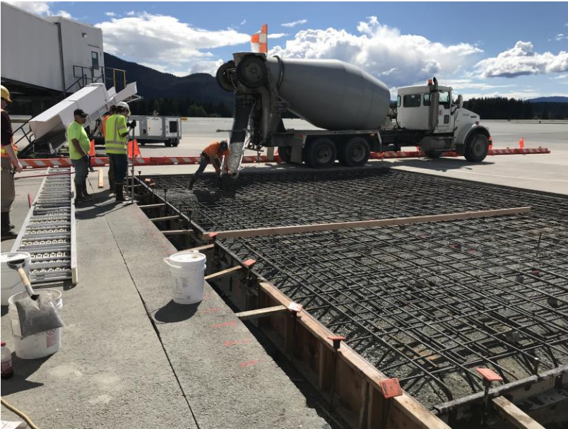
Concrete placement begins at Gate 2 expanded hardstand.
