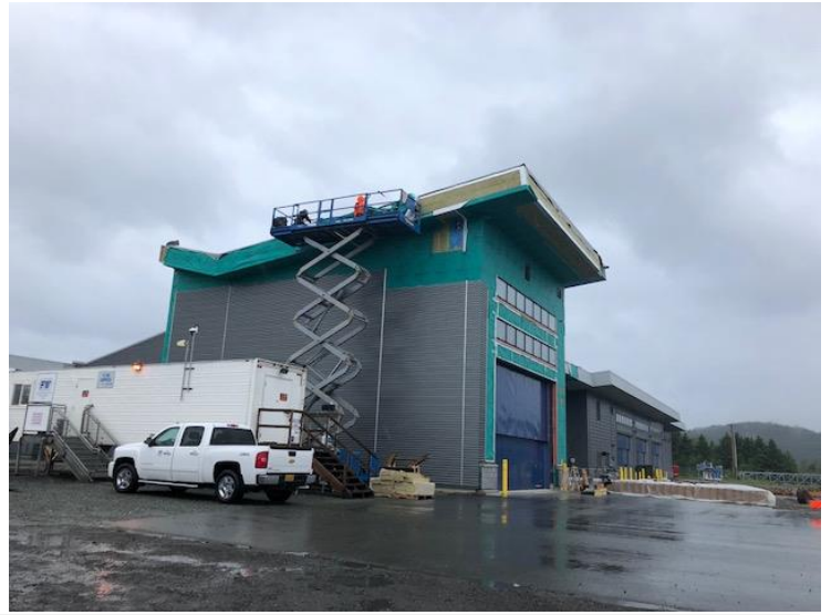
SREB exterior doors painted, and east wall of maintenance bay receives siding (wash bay reclamation pit formwork at right).
