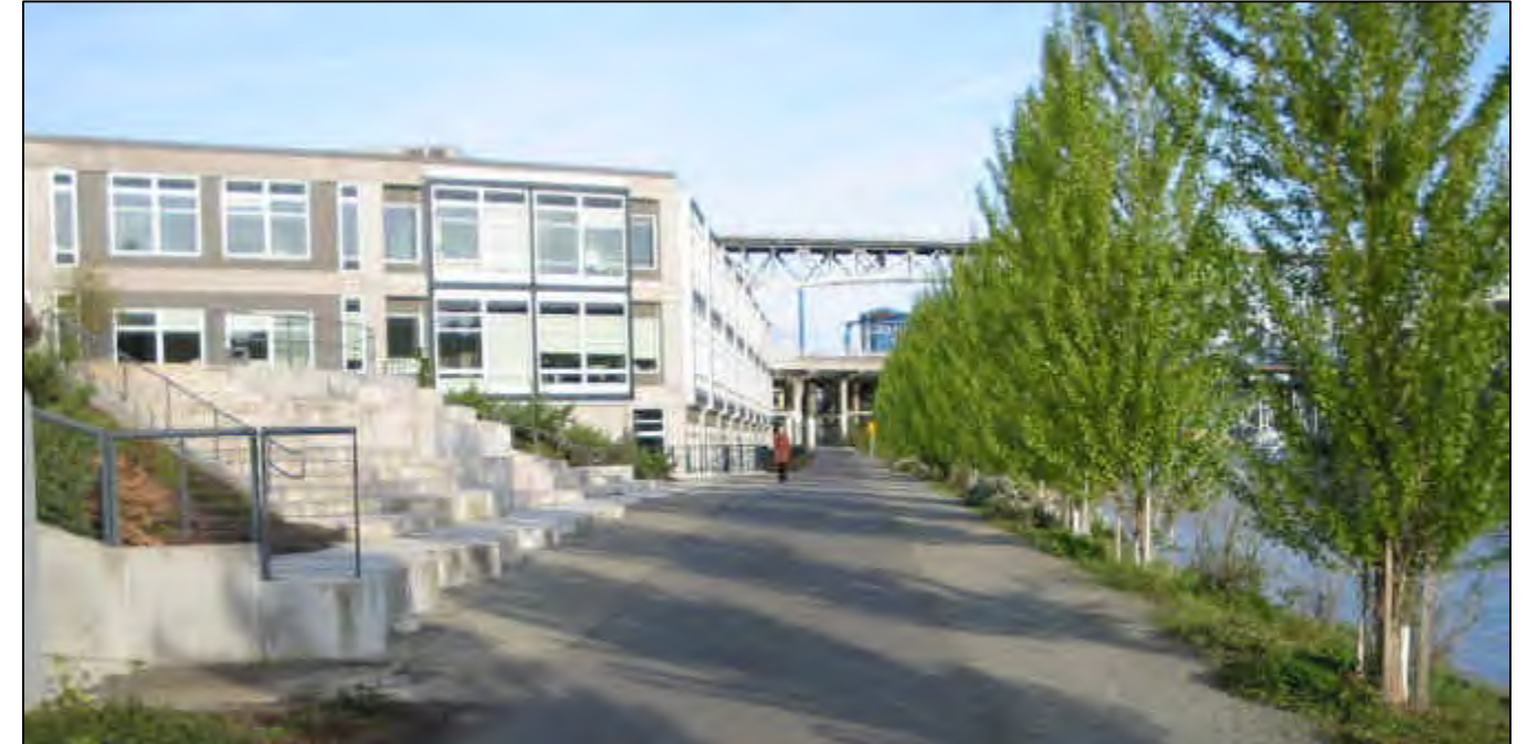
View of Similar Waterside Massing and Scale Treatments (Area A)
