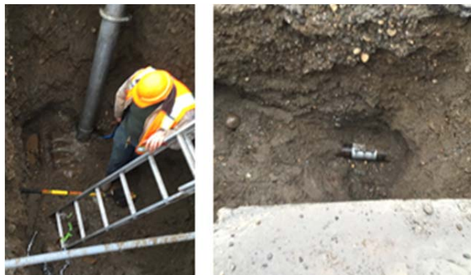
Valley Court mainline leak located and repair sleeve installed
