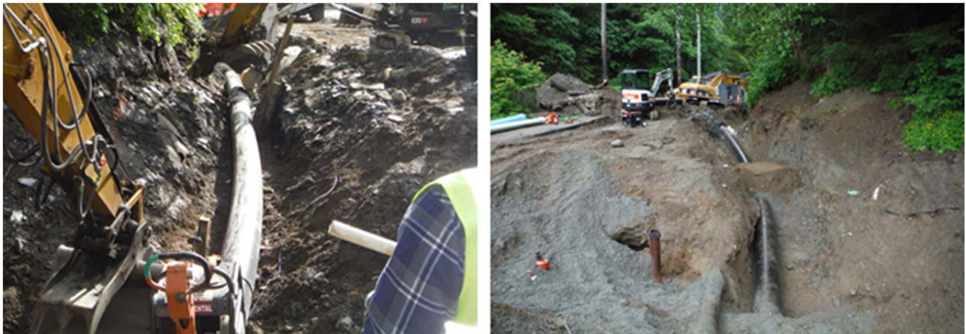
HDPE waterline installation at Cope Park
