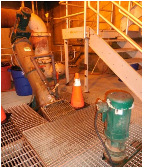
Left to right: MTP existing screening (equipment to be upgraded); JDTP existing influent channel (to be abandoned)
