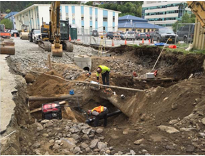
HDPE waterline installation on Whittier Street
