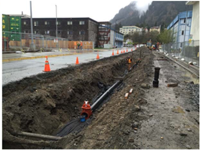
HDPE waterline installation on Whittier Street
