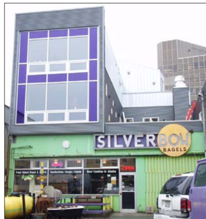
An appropriate rear-facing alley addition.
