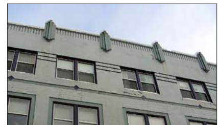
Cornice details in Juneau's Downtown Historic District.
