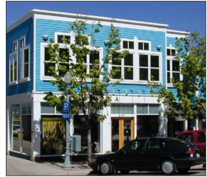
Example of new construction which would relate to existing historic structures by maintaining the alignment of horizontal features, producing a similar floor to floor height, dividing a larger facade into smaller modules and maintaining the visual scale of buildings. (Aspen, CO)
