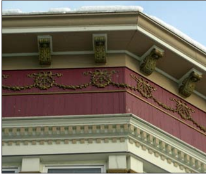
Projecting parapet caps with elaborate supporting bracket work can be seen in this cornice detail. Below the brackets, a strand of decorative metalwork laces the building.
