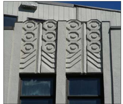
Geometric shapes enrich cornices and other facade components in the Art Deco style.
