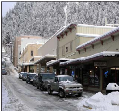
Canopies step with the street level.
