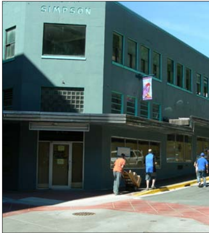
A clearly defined entry is commonly covered by a canopy.
