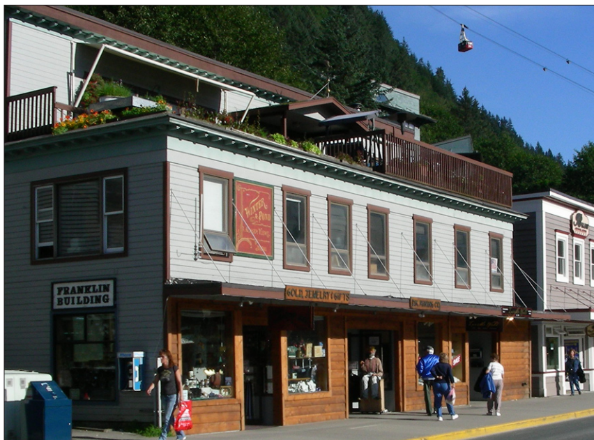
The Madsen's Rooming House (1899, 369 S. Franklin Street) is a contributing structure. The storefront material is a later alteration that detracts. A more appropriate material should match the historic profile and be painted.
