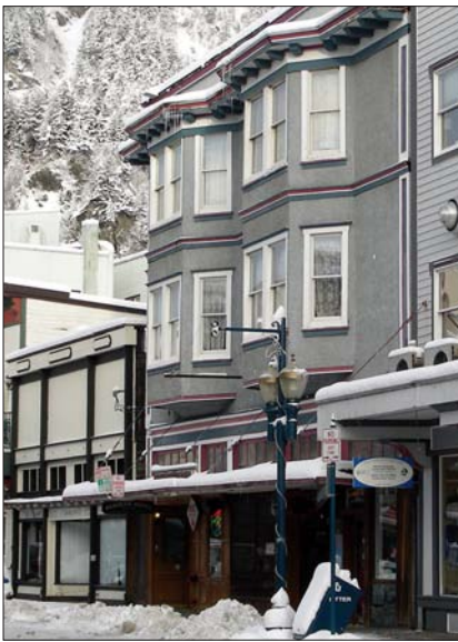
The addition of a canopy is visible in these photographs from 1913 and 2006. The canopy was added during the historic period.
