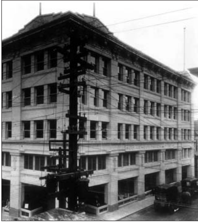
Characteristics of the Early 20th Century Commercial Style, such as a corner recessed entry, concrete construction and rectangular fenestration patterns, can be found in the Goldstein Building (1914, 130 Seward Street).
