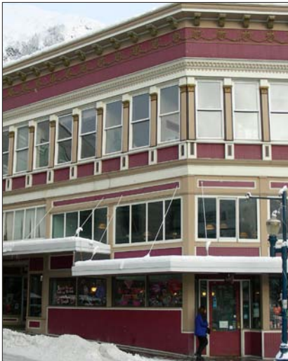
Projecting parapet caps with elaborate supporting bracket work can be seen in this cornice detail. Below the brackets, a strand of decorative metalwork laces the building.
