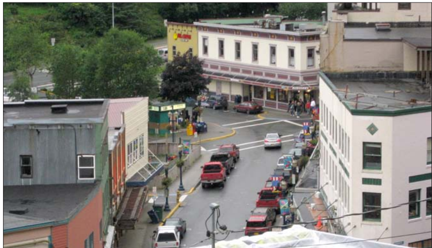
Flat roofs are the most common roof form in Downtown Juneau.
