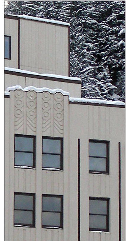
Concrete and masonry features shall be preserved.
