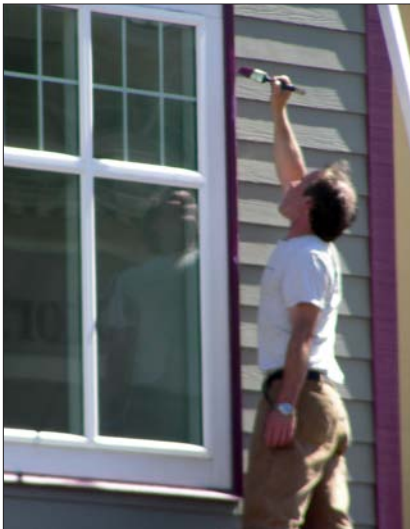
One or two paint colors are generally used as accents over one background color which unifies the typical painting scheme of historic buildings in Downtown Juneau.
