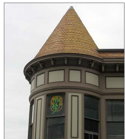
In-kind replacement, as seen on the roof shingles above in 2007, is an option.
