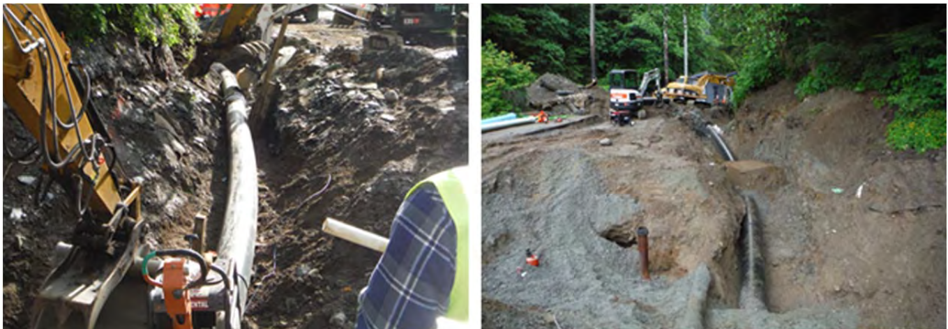
HDPE waterline installation at Cope Park
