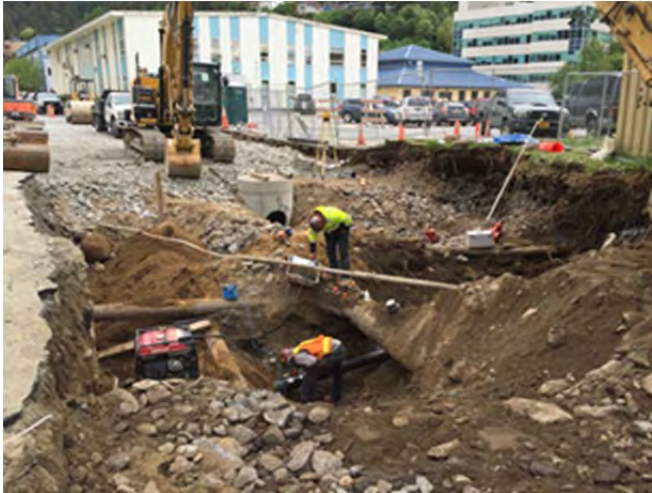
HDPE waterline installation on Whittier Street
