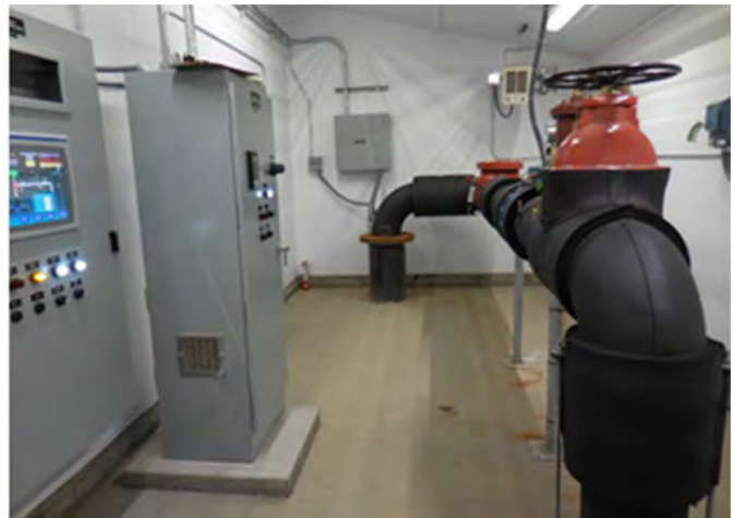
New well house, pumps, piping and controls in well house at LCB
