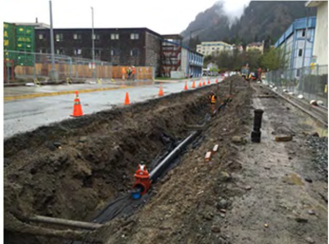
HDPE waterline installation on Whittier Street
