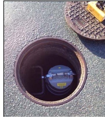
Photo of sampler inside a manhole.
