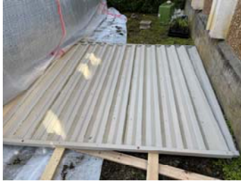
Typical siding panel. Siding panels were ganged together and installed in large sections with exposed fasteners through face and perimeter trim.
