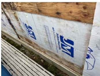
View of polyiso insulation behind plywood substrate at base of wall.
