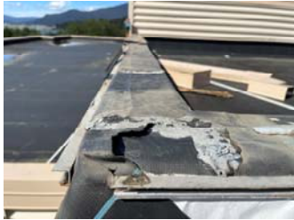
EPDM membrane corner above the southwest corner of storefront and composite metal panel siding. The EPDM is missing seam tape and the membrane lap is open which could allow water to infiltrate into the wall under the metal parapet cap flashings.
