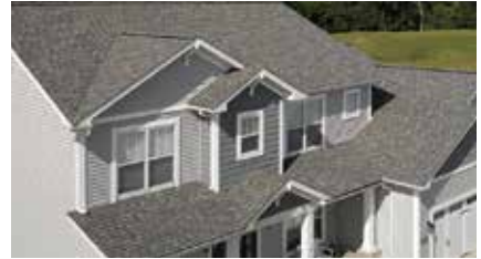
ROOFING AND VENTILATION
