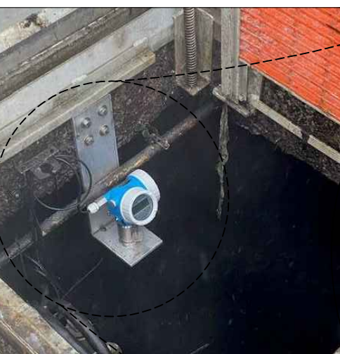
1 OD WET WELL HATCH MODIFICATION & INSTRUMENTATION INSTALLATION S-101 NTS
