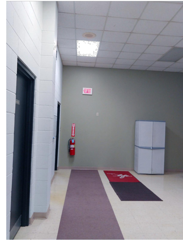
3 PHOTO - MAIN CORRIDOR 201 NO SCALE
