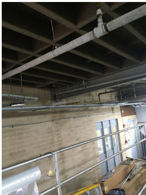
4 PHOTO - HEADWORKS SPACE NO SCALE
