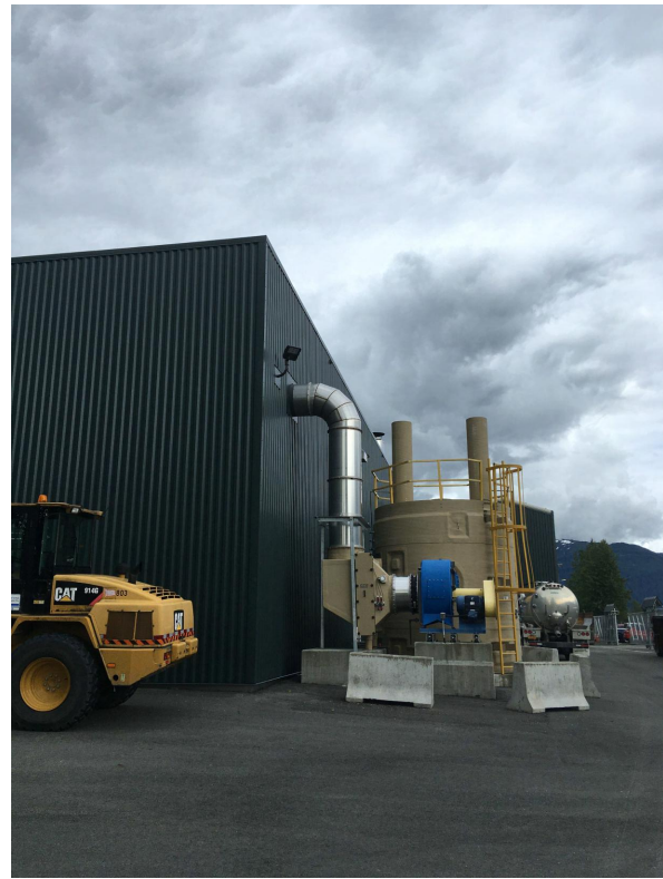
1 PHOTO - BIO SOLIDS EXTERIOR NO SCALE
