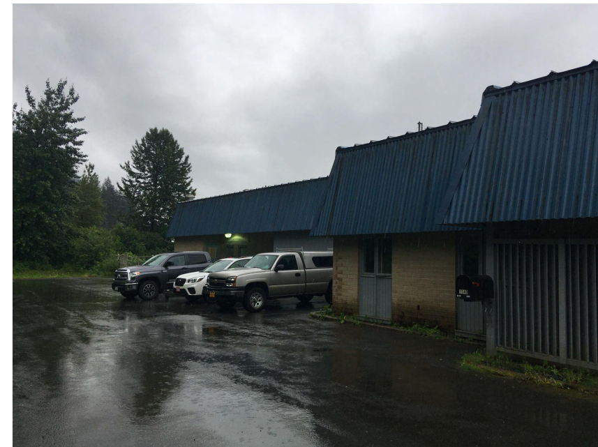
3 PHOTO - CONTROL BUILDING EXTERIOR NO SCALE
