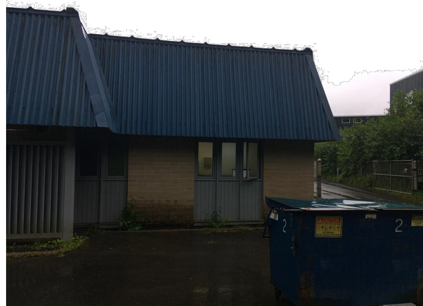
2 PHOTO - CONTROL BUILDING EXTERIOR NO SCALE
