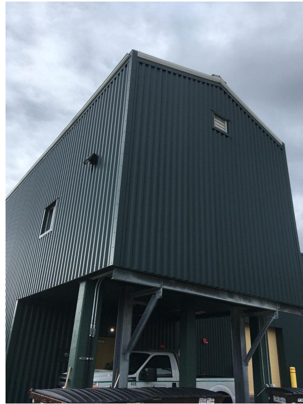
2 PHOTO - BIO SOLIDS EXTERIOR NO SCALE
