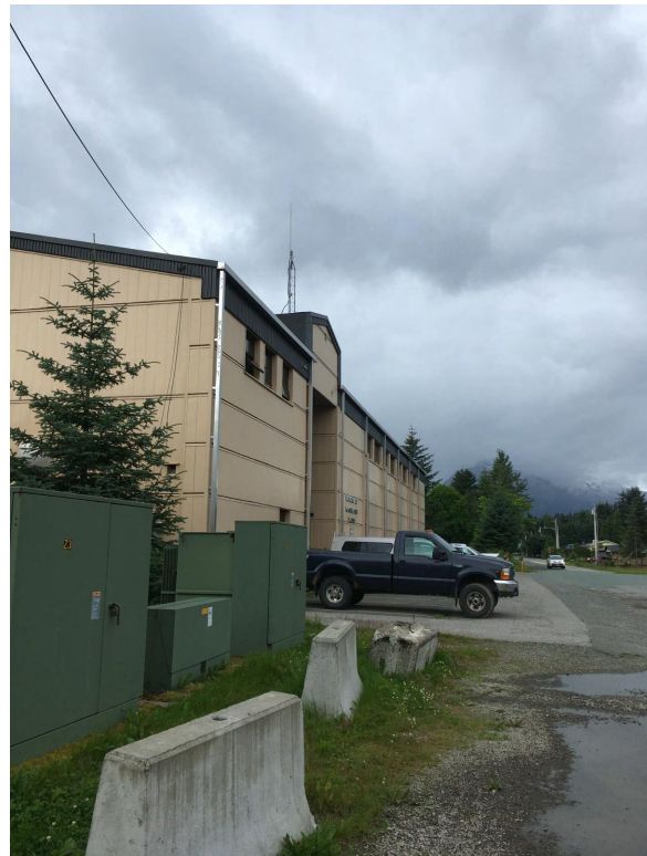
1 PHOTO - SBR EXTERIOR NO SCALE
