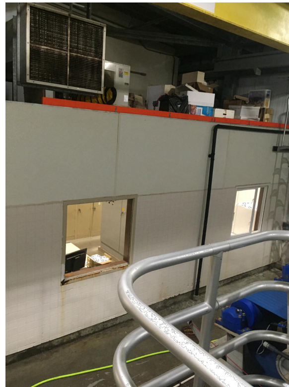
2 PHOTO - CONTROL ROOM NO SCALE
