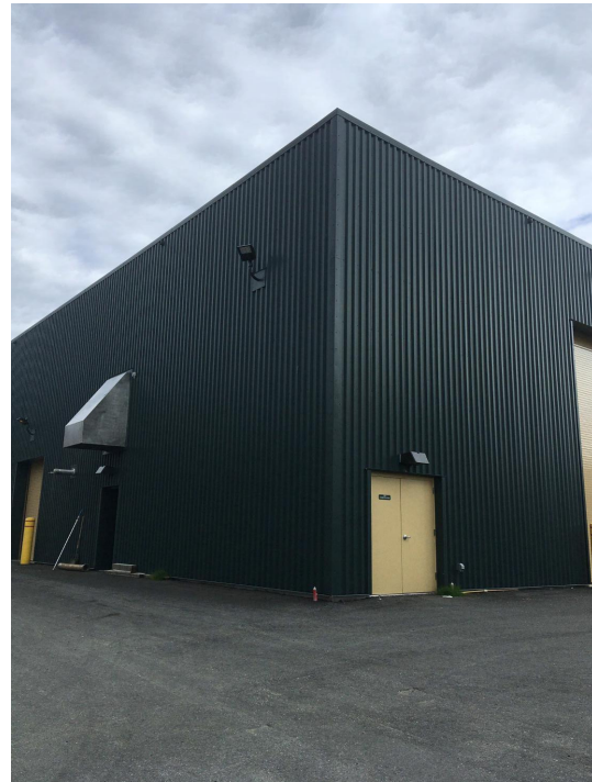
4 PHOTO - BIO SOLIDS EXTERIOR NO SCALE
