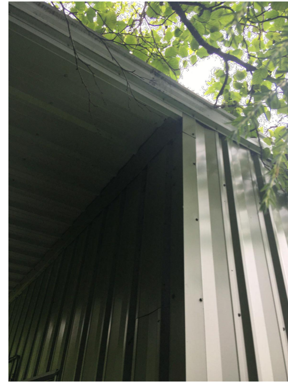
3 PHOTO - BUILDING EXTERIOR NO SCALE
