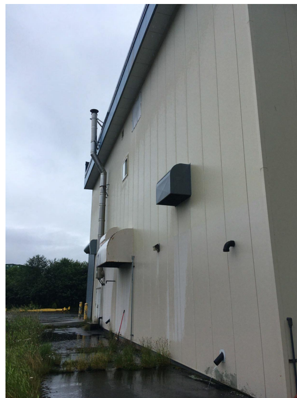
5 PHOTO - INCINERATOR BUILDING EXTERIOR NO SCALE
