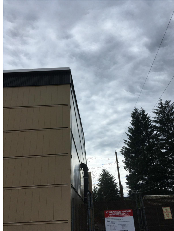
2 PHOTO - SBR EXTERIOR NO SCALE
