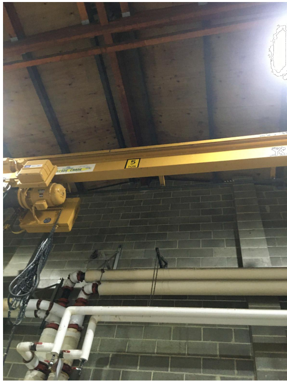
1 PHOTO - BLOWER ROOM 218 NO SCALE
