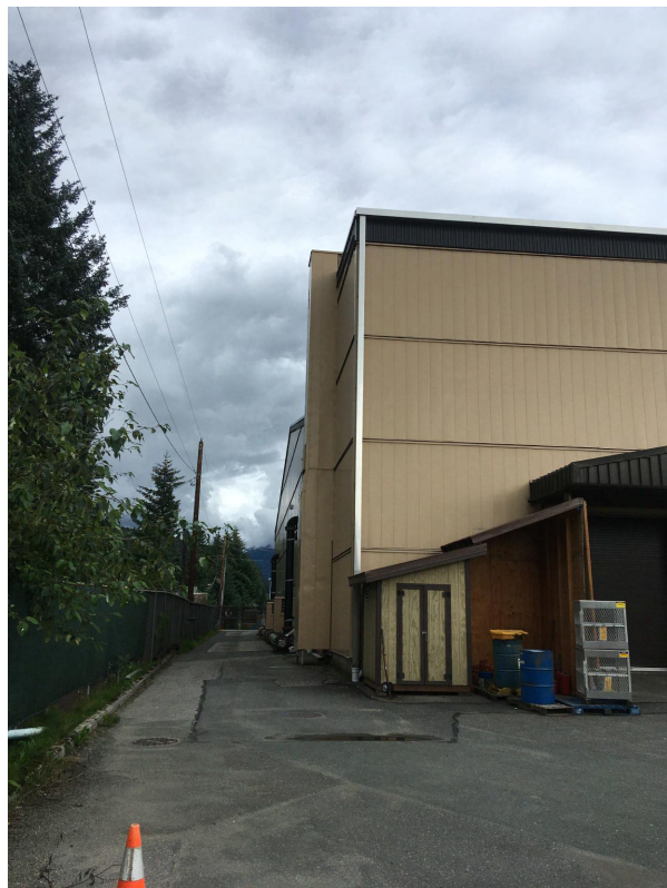
4 PHOTO - SBR EXTERIOR NO SCALE
