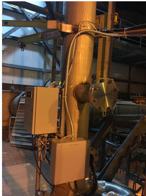
1 PHOTO - RADIO TERMINAL UNIT NO SCALE
