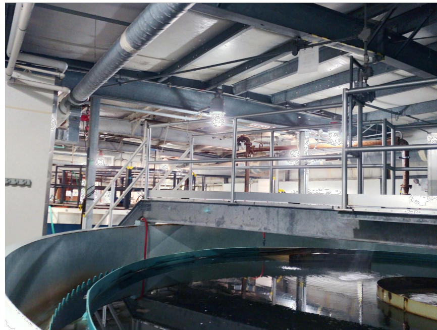
5 PHOTO - BUILDING INTERIOR NO SCALE
