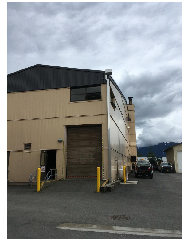
6 PHOTO - SBR EXTERIOR NO SCALE
