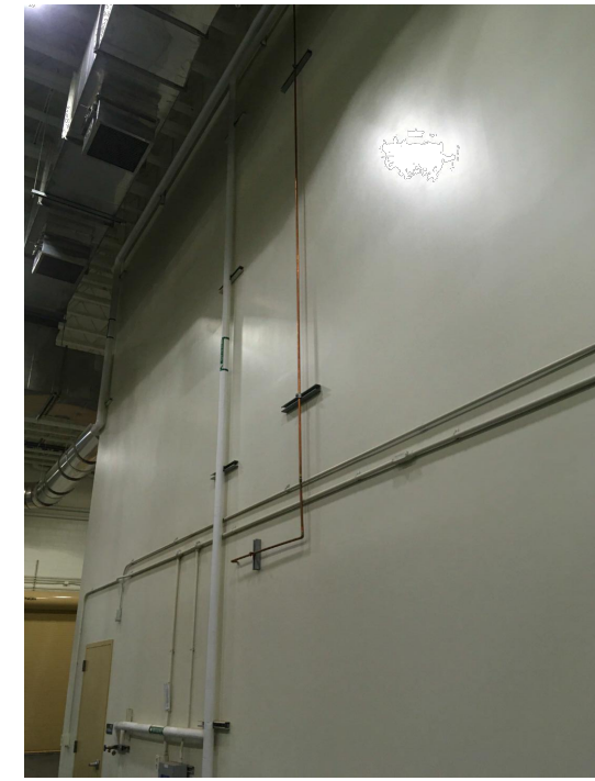
3 PHOTO - DRYER ROOM 101 NO SCALE
