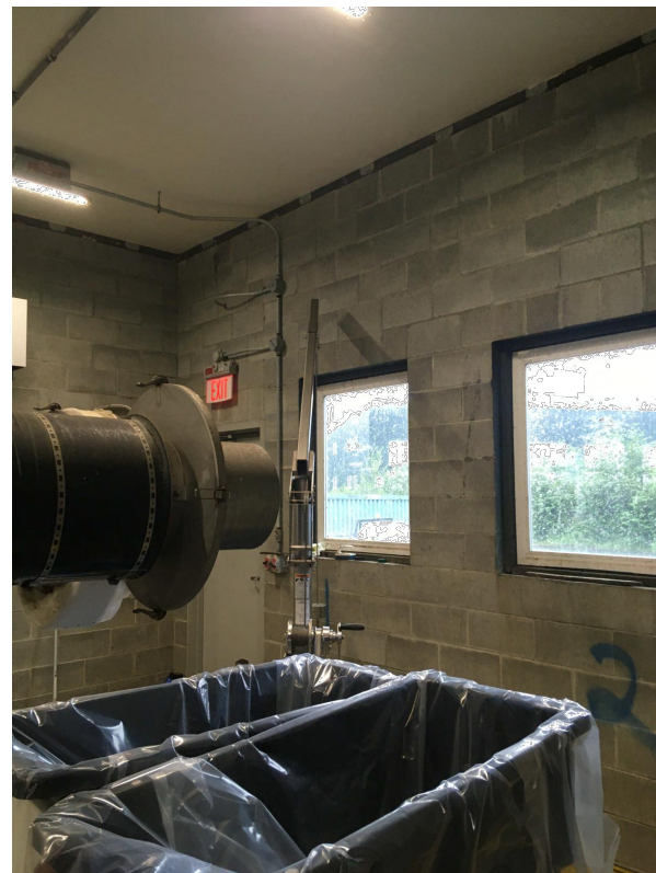
5 PHOTO - HEADWORKS SPACE NO SCALE
