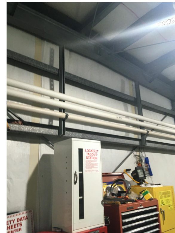
6 PHOTO - BUILDING INTERIOR NO SCALE
