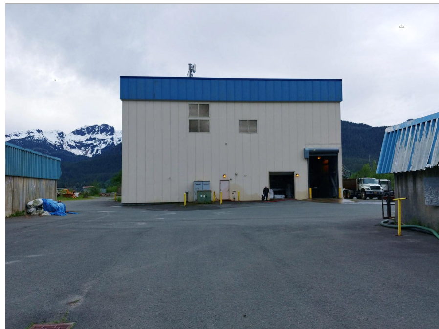
4 PHOTO - INCINERATOR BUILDING EXTERIOR NO SCALE
