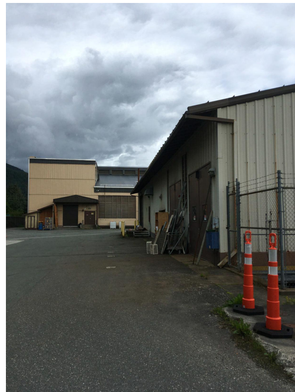
5 PHOTO - UV BUILDING EXTERIOR NO SCALE
