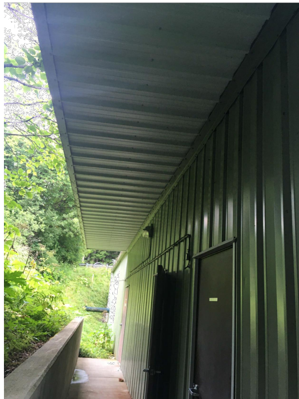
4 PHOTO - BUILDING EXTERIOR NO SCALE
