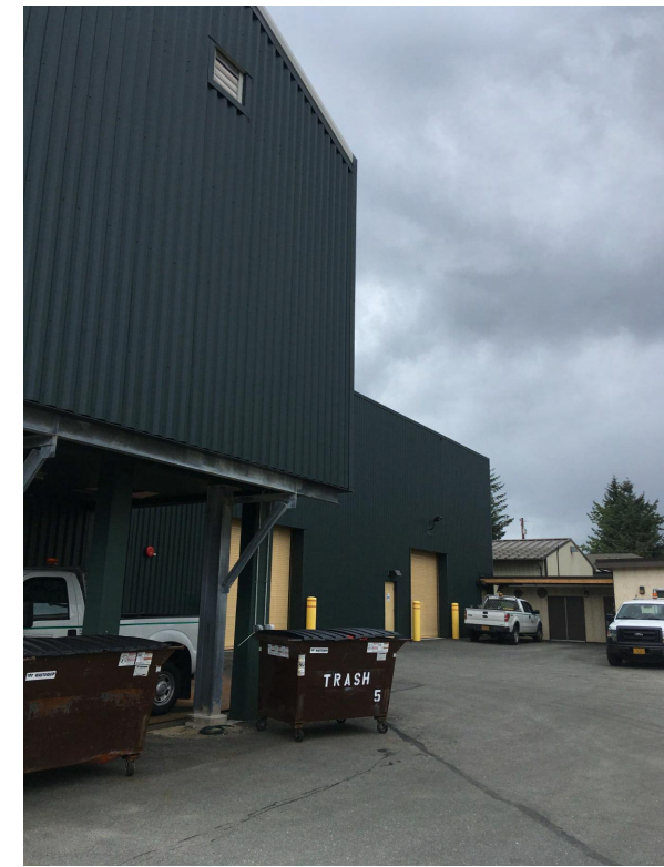
3 PHOTO - BIO SOLIDS EXTERIOR NO SCALE
