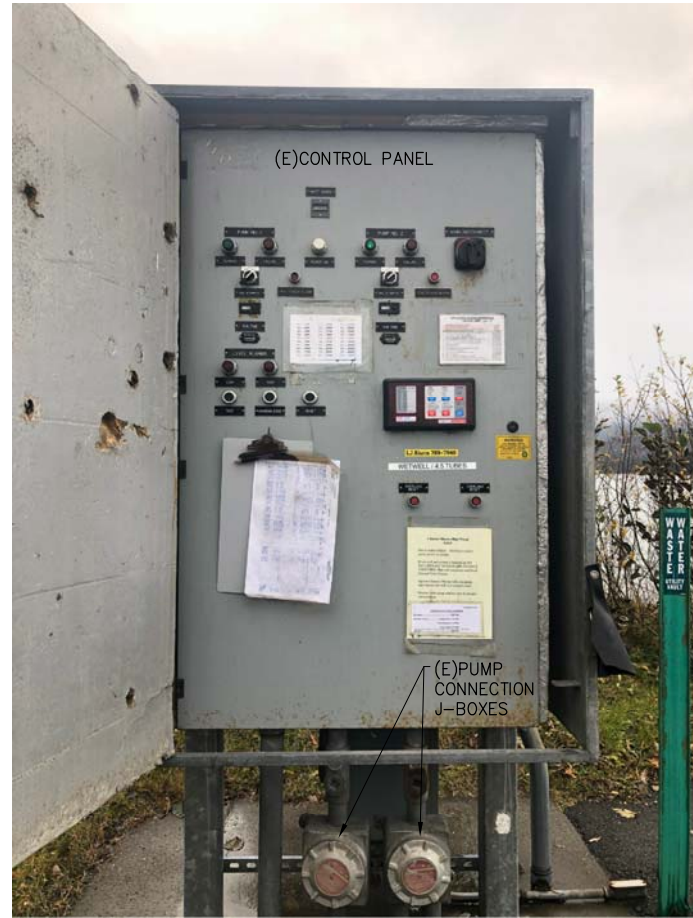
2 CHANNEL DRIVE - (E) CONTROL PANEL DEMOLITION E9
