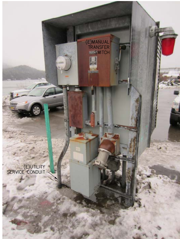
1 CHANNEL DRIVE - (E) POWER DEMOLITION E9
