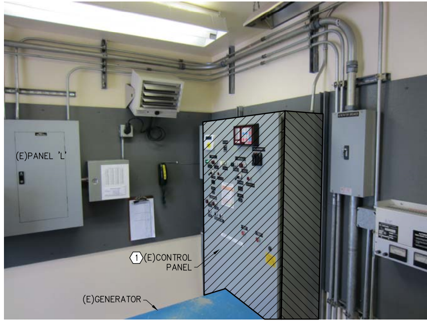
1 CHANNEL VISTA GENERATOR BUILDING - DEMOLITION PHOTO E12
