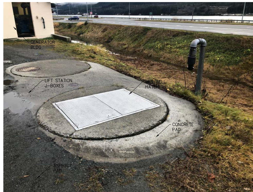
5 (E) WET WELL / VALVE VAULT LAYOUT E17
