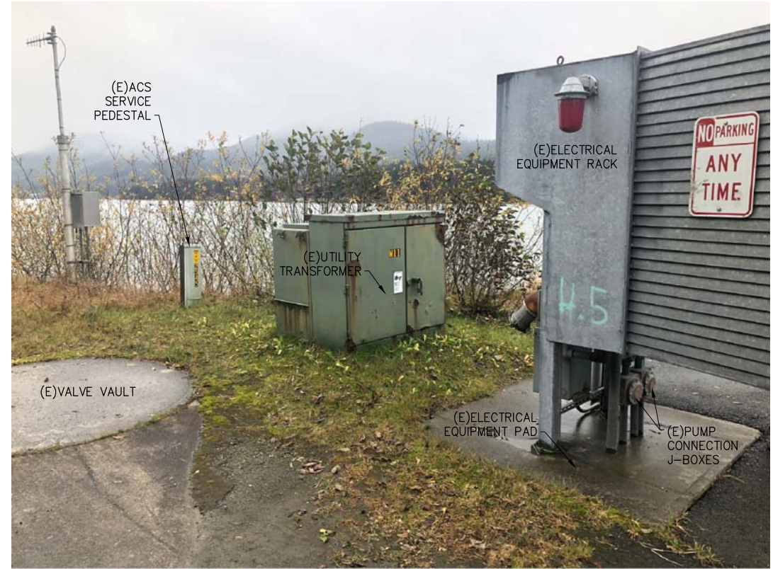
3 CHANNEL DRIVE - SITE ELECTRICAL DEMOLITION E9
