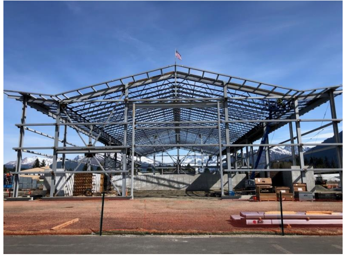
Sand/Chem Building: Steel complete; roof decking begins along east side.
