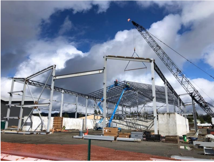
Sand/Chem Building: Steel erection, view from Southeast corner.
