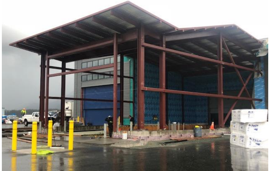
North elevation of SREB Wash Bay.
