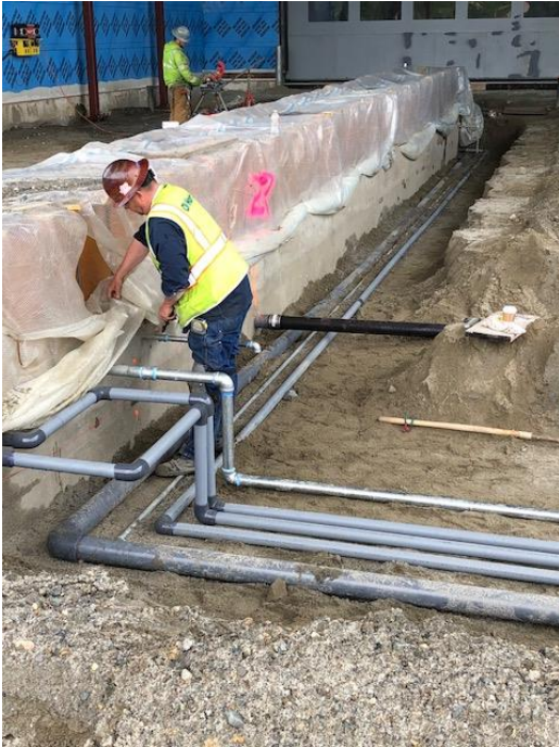
Installation of underground piping at SREB Wash Bay.
