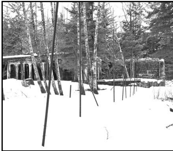
Tennis Court Posts in Foreground--Central Steam Plant in the background MLKing 2007
