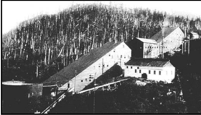
Cyanide Plant and Refinery for Producing Gold Bars AEL&P
